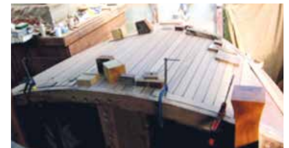
6mm Teak deck planks were laid over marine ply.
