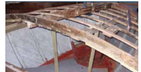
New aft deck under construction.
