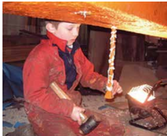
Installing the new ones.
