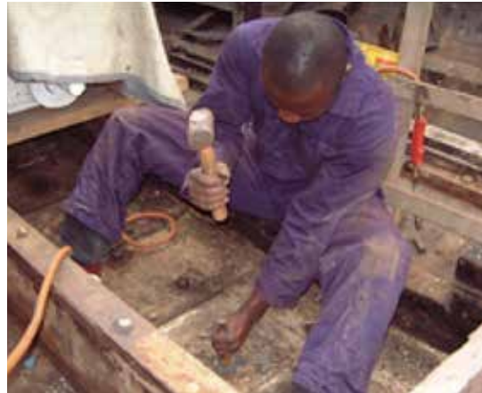
Driving out the old bolts.
