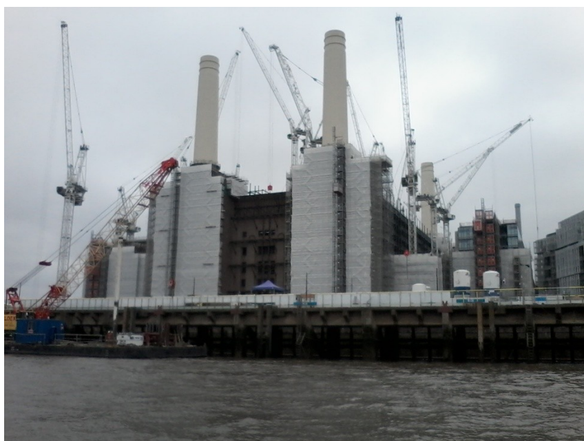
Battersea power station with cranes everywhere
