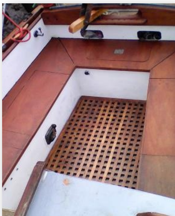
The new cockpit, sides, and some coaming replaced and new seats
