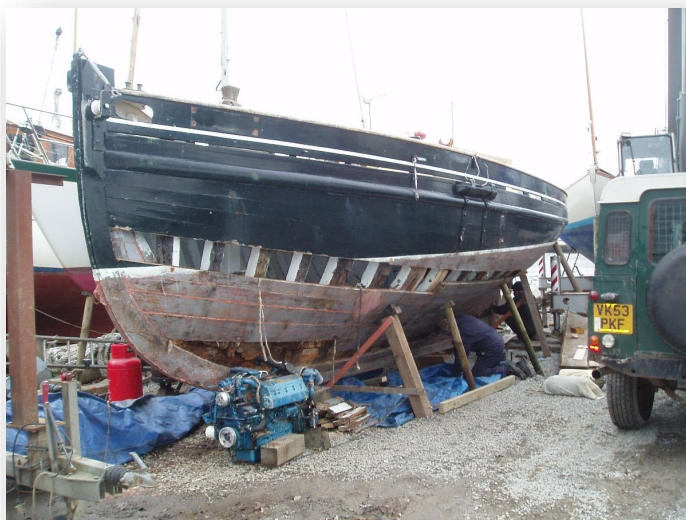
Restoration of Wanderer 11
