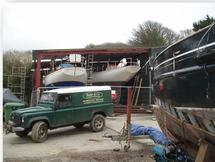
New storage shed nearing completion photos: Ashley Butler
