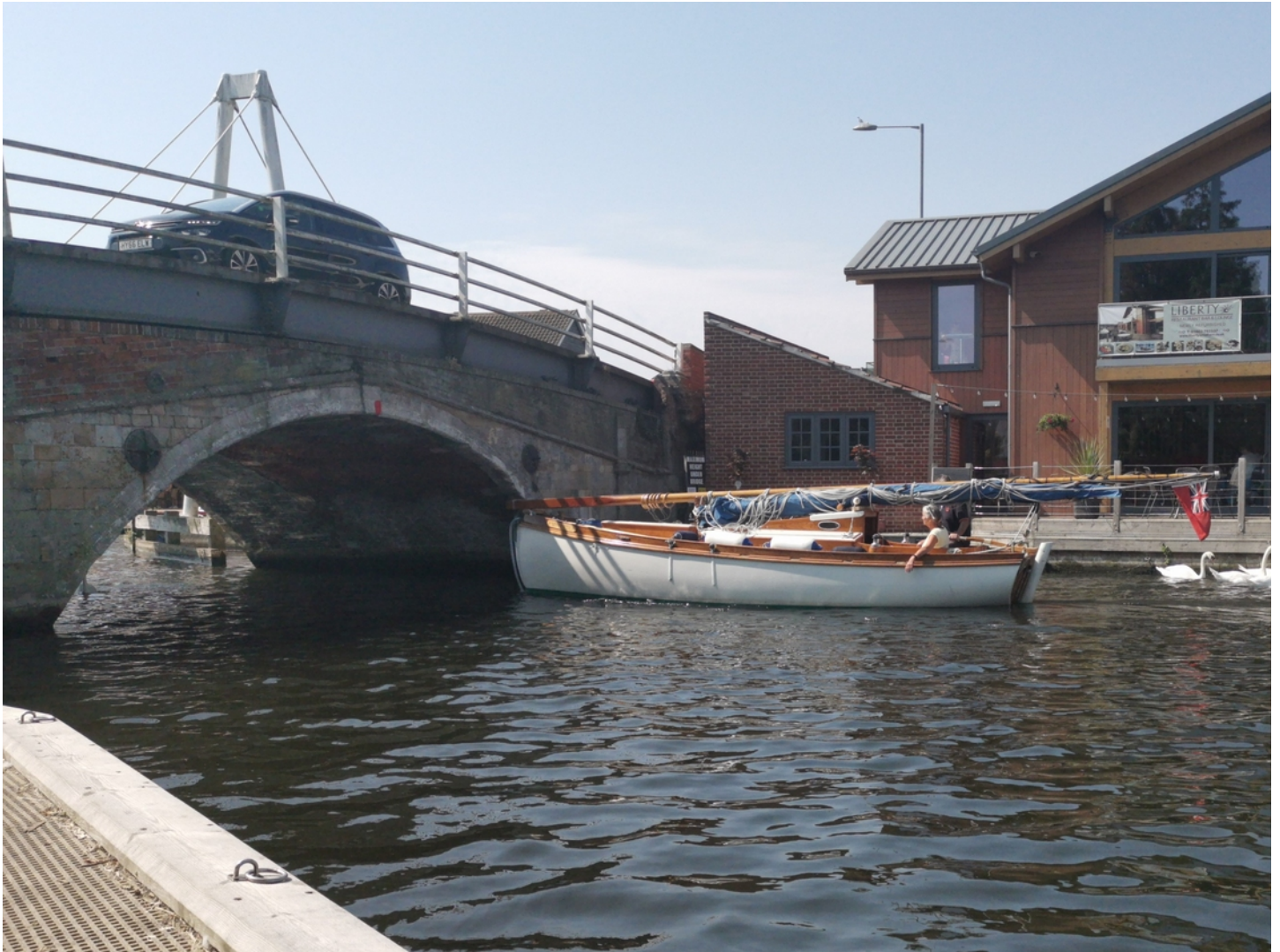
Going through Wroxham Bridge
