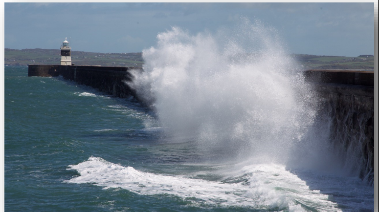
The breakwater at Holyhead all astir
